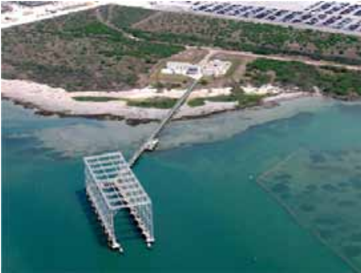
The Electromagnetic Reduction (EMR) facility is a focal point for the redevelopment strategy of Naval Station Ingleside.
